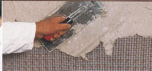
Simply lay on plaster with a trowel.
