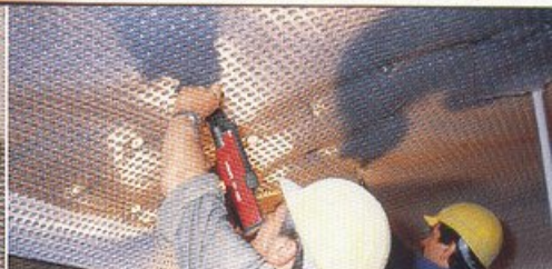
In tunnels, DELTA®-PT supports shotcrete applications.
