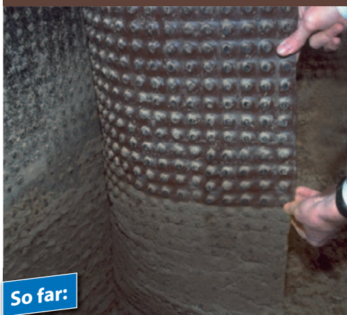
The dimples of many dimpled sheets press against the bitumen coating of cellar walls – a severe stress on the waterproofing.
