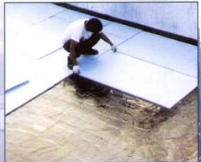
INSULATION TO CONCRETE ROOF
