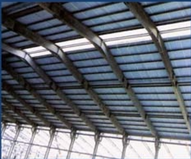
INSULATION TO METAL ROOF
