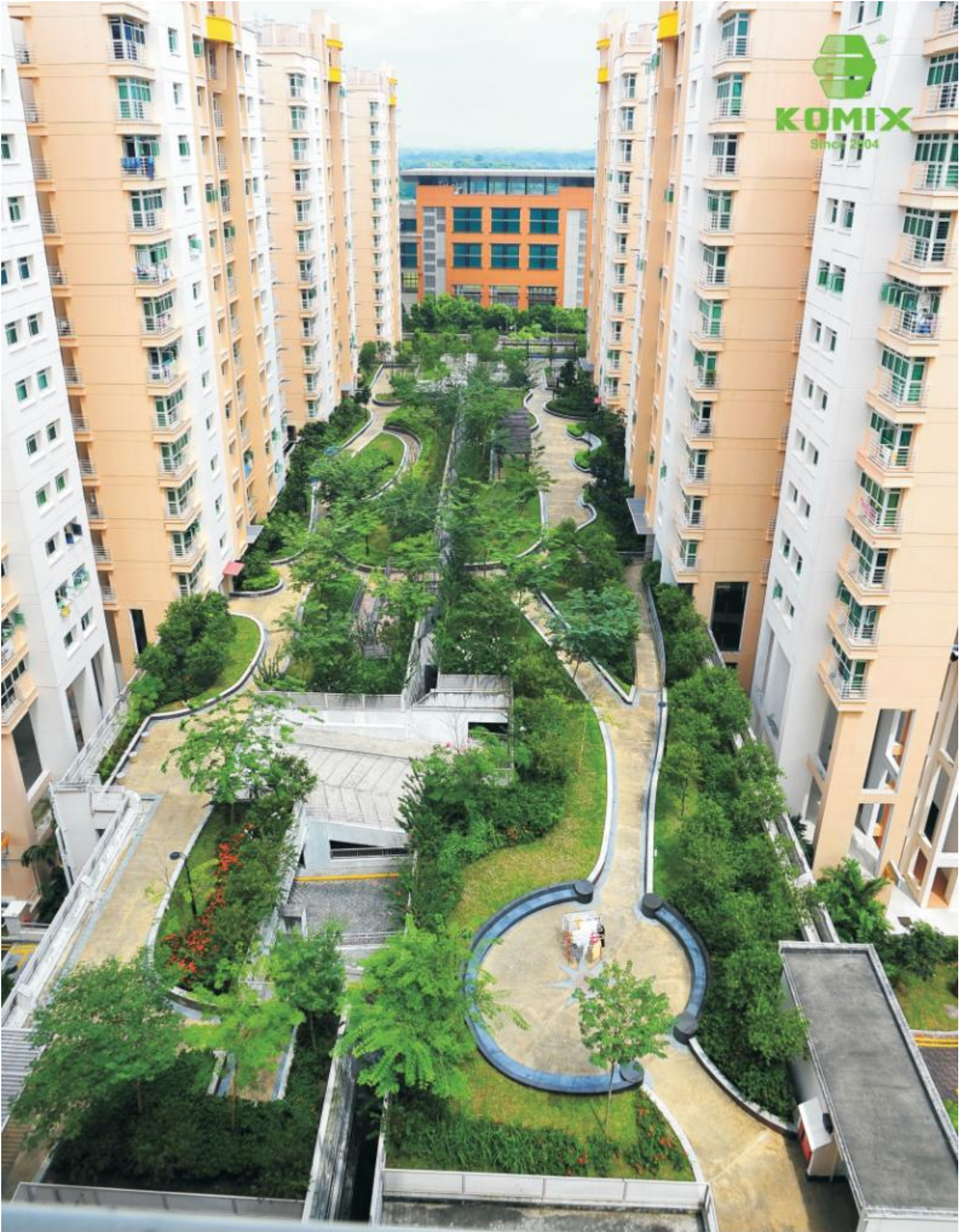
HDB Car Park, Blk 171 Punggol Field, Singapore
